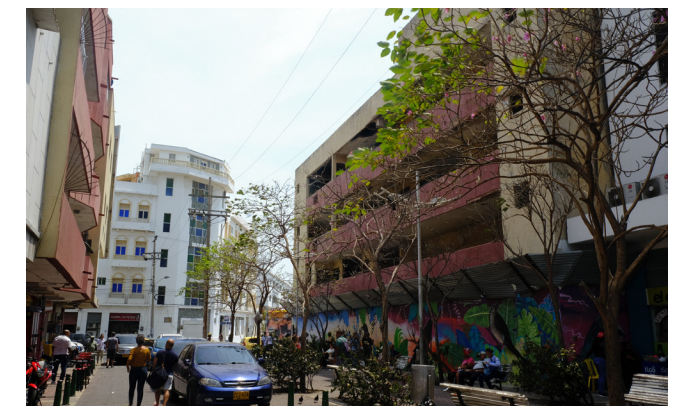
Figure 8.7 – Example of building suitable for strategic rehabilitation Photo: Laura Margaret Sollmann, Sung, Di
